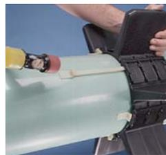
6. Insert all Slide-Locks as far as possible by hand. Complete tightening by tapping each Slide-Lock with a hammer, while holding the Slide-Lock against the pipe.
