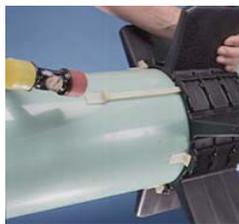
7B. Re-insert Slide-Locks into segments or until tight by driving Slide-Lock back into position while holding the Slide-Lock against the pipe.
