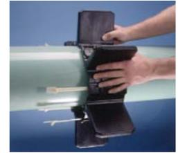
5. Align the buckles and lock into place. Take the final Slide-Lock and slide into place.
